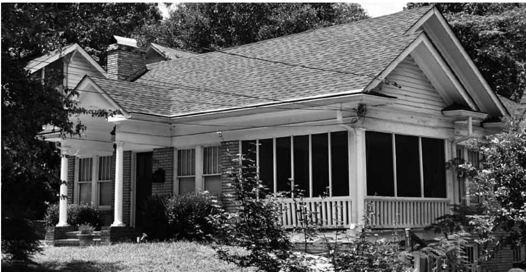
In 1923, the city of Atlanta selected the home located at 57 Orme Circle as a “demonstration house” for the Better Homes Movement. This home sits on the lot today (now 562 Orme Circle).
